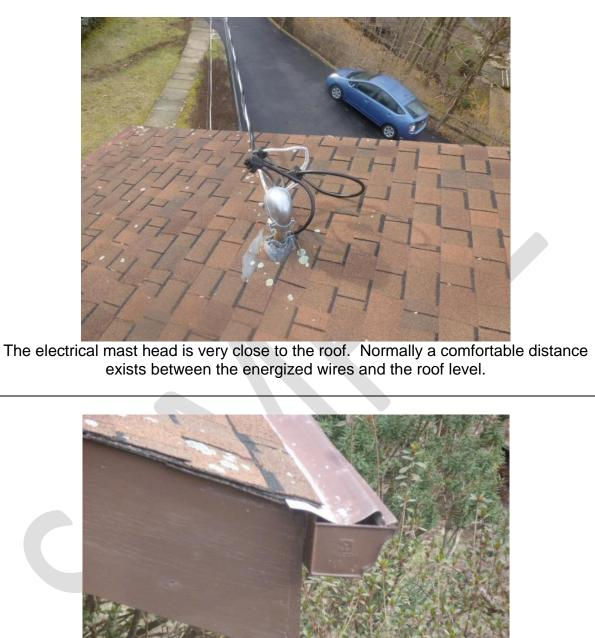
An ill-fitting gutter cover is in place. It is improperly installed and must be corrected or replaced with a suitable cover
